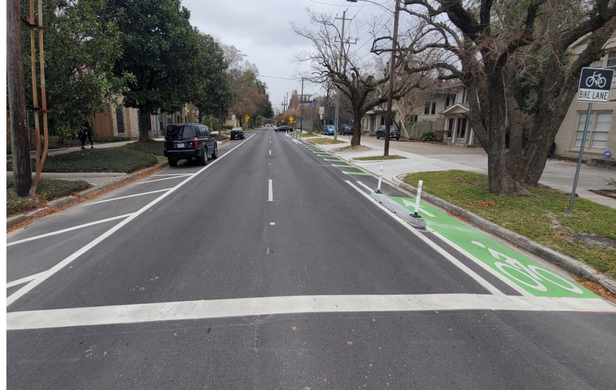
After Construction Commonwealth. South of Welch St
